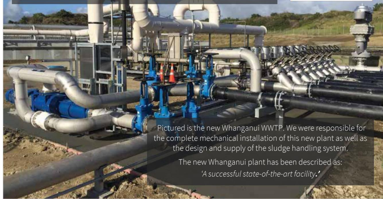
Pictured is the new Whanganui WWTP. We were responsible for the complete mechanical installation of this new plant as well as the design and supply of the sludge handling system.
